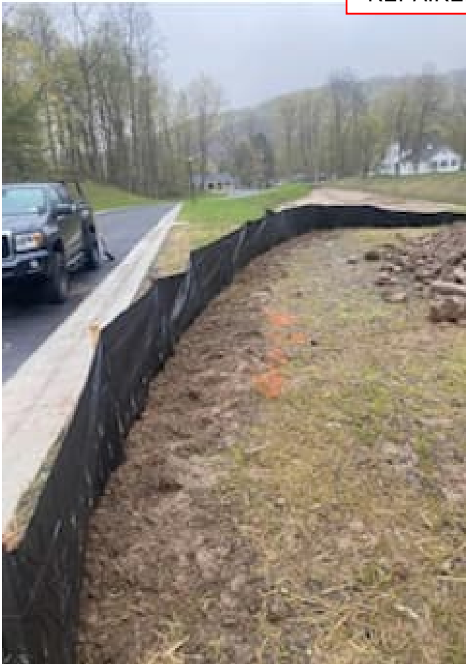
**REPAIRED SILT FENCE
