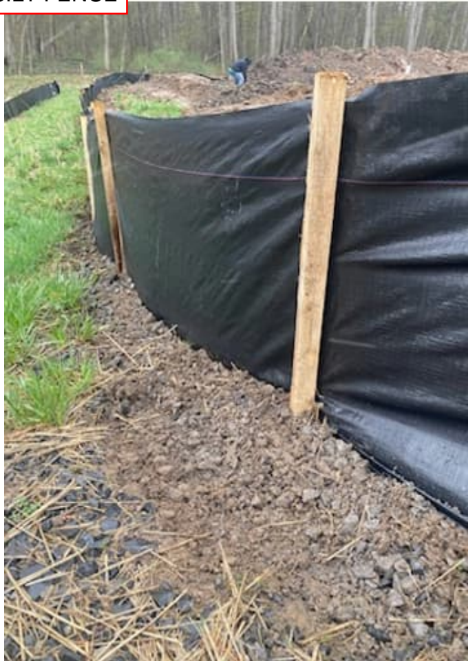
**REPAIRED SILT FENCE
